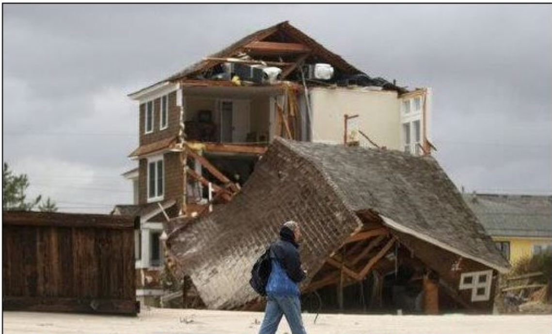
Image #8: The above example photo illustrates a building that is split/sheared.
